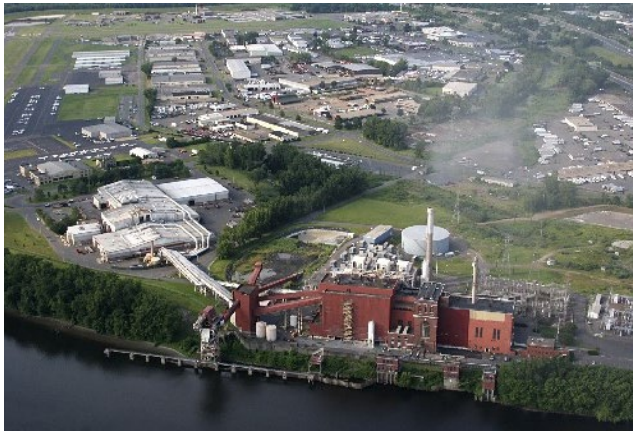
MIRA Hartford Incinerator
