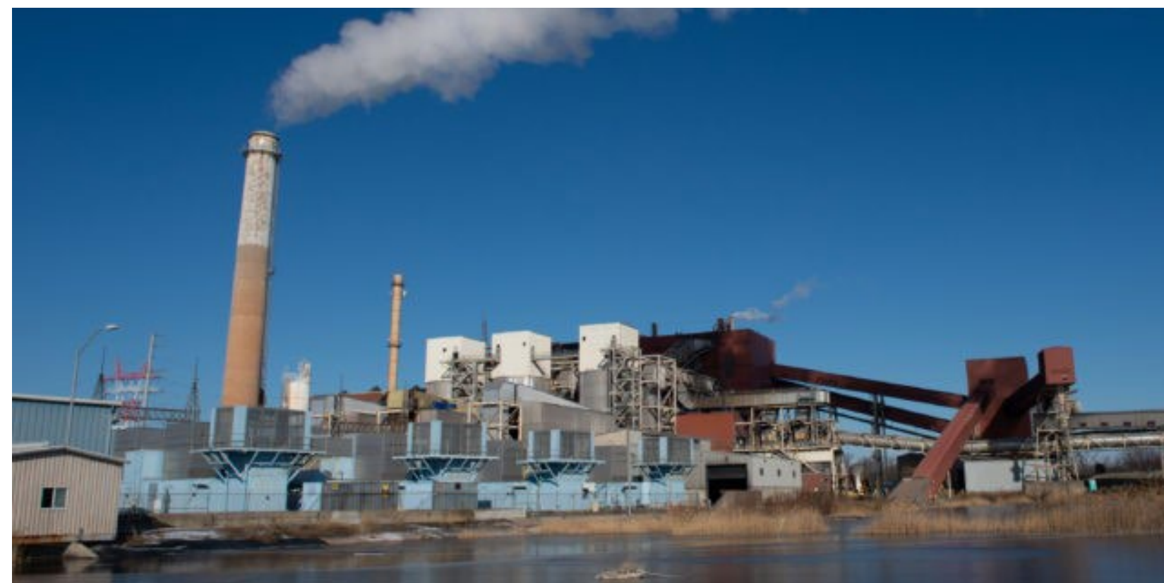
MIRA Hartford Incinerator
