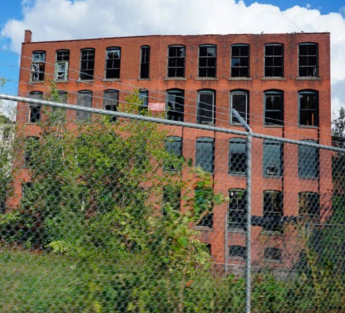
Waterbury Companies, Inc. - 835 South Main Street, Waterbury
